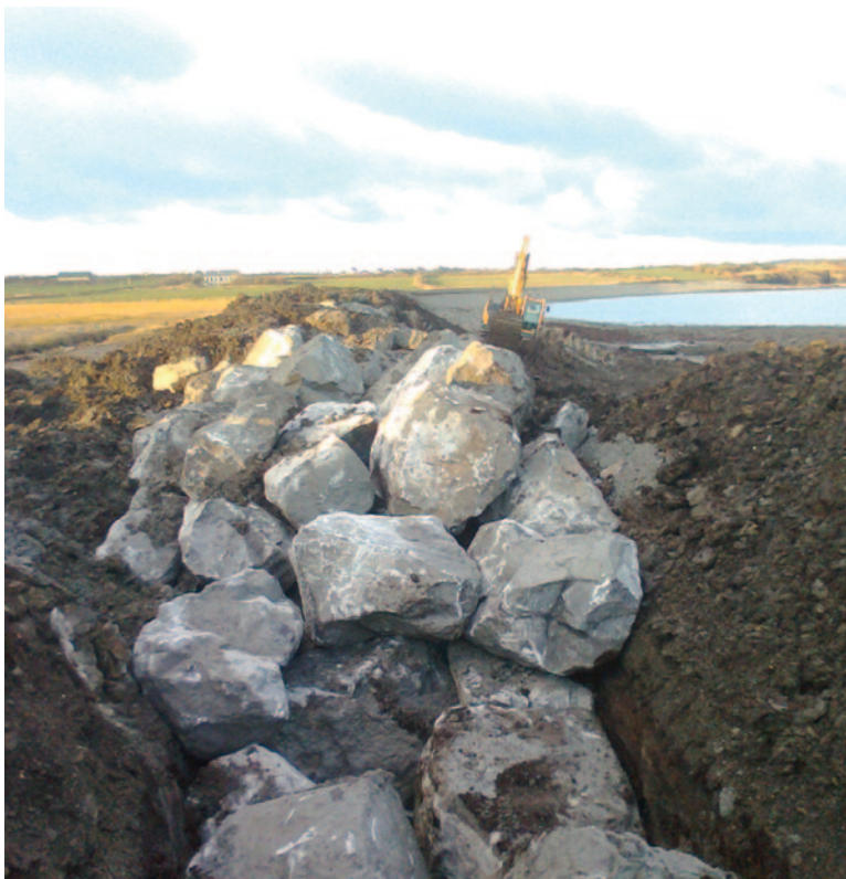
Construction of rock armour wall, Kilcredaun, Co. Clare.
